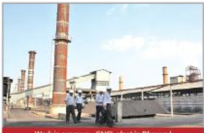
Work in progress - GNCL plant in Dharwad
